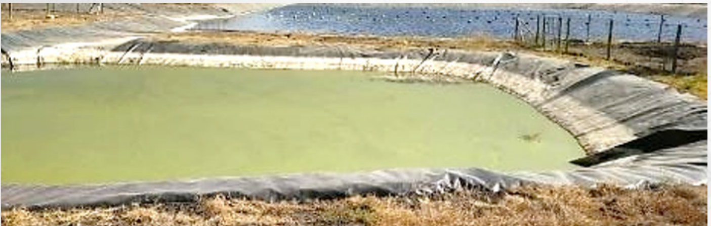
The dam in the front receives all stormwater and treated waste water from the wetlands. Once solids have settled, clear water is pumped to the irrigation dam at the back.
