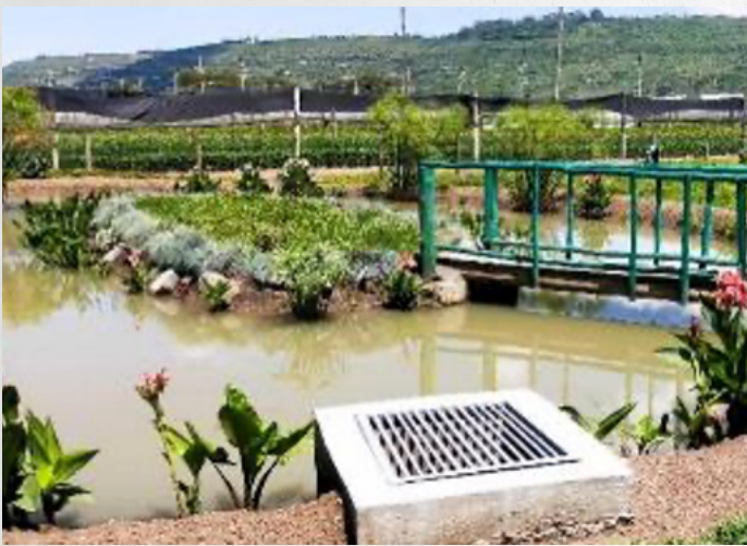
A newly constructed wetland pond on Kariki Naivasha farm. The maintenance hole offers a bypass from one pond to another (e.g. from 1 to 3 when pond 2 is undergoing routine maintenance).
