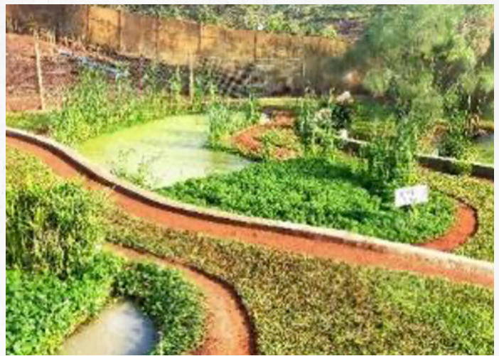
A good view of the series of newly constructed and planted wetland ponds on Kariki KR farm (Thika).
